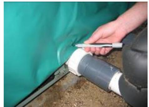
3. Using a marker pen, mark the height and position of the flow and return pipes on the cover
